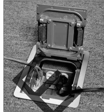
Cellular Metal Floor Raceway
